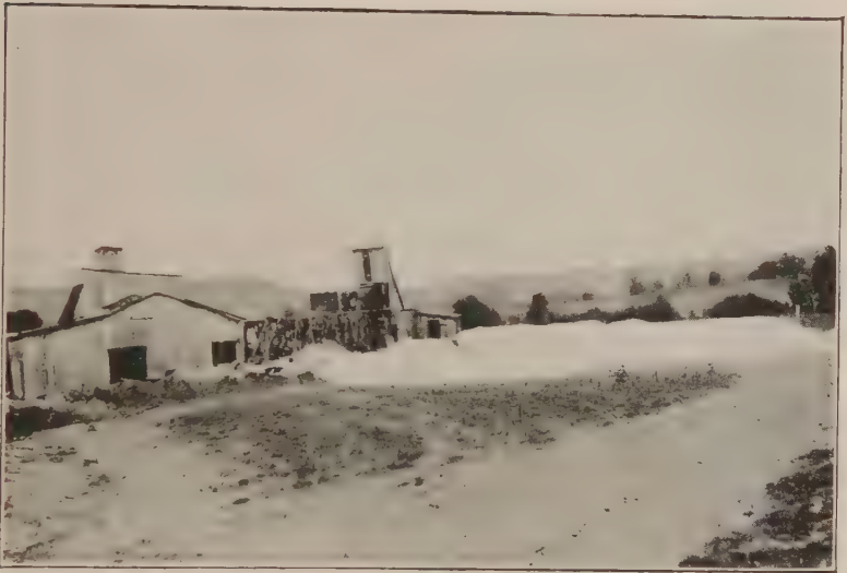
(21) Surface plant at Liberty Bond mine, Salem district.
